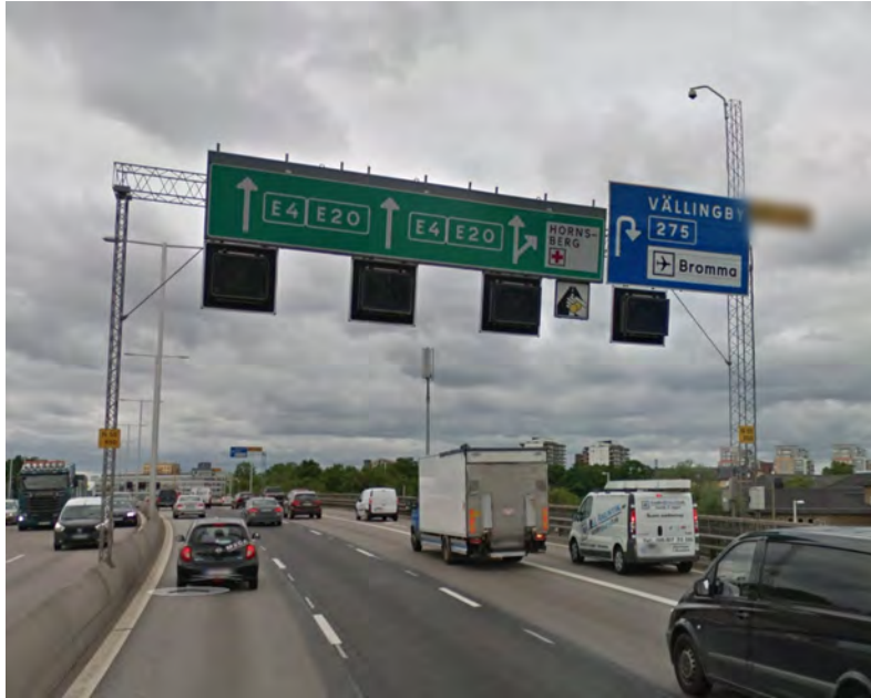
Figure 1.2: A sensor array. This one is located on E4N at kilometer reference 55650, as can be seen on the yellow signs. The sensor furthest to the right has lane ID 1, the sensor next to it lane ID 2, and so on. Picture taken from Google Maps' street view.
